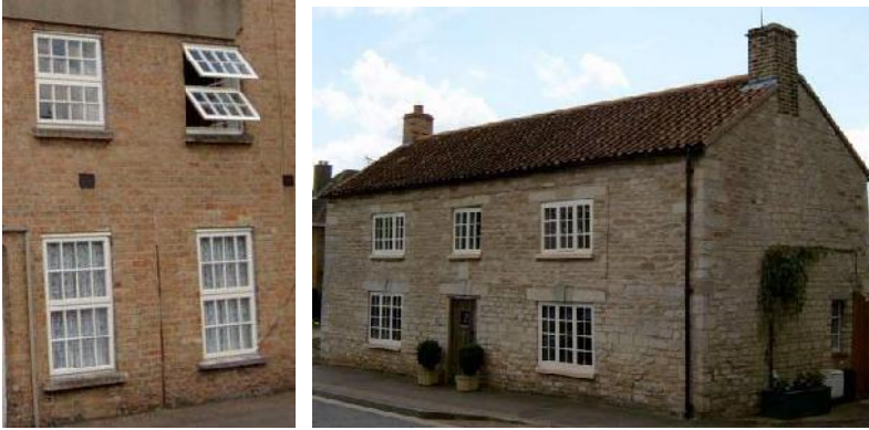
20th c. sash and casement replacement windows.
