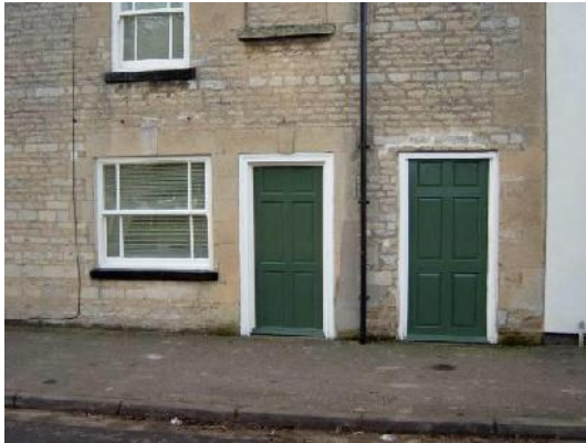
19 th c. doors & windows replaced in replica
