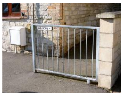
Modern utilitarian railings.
