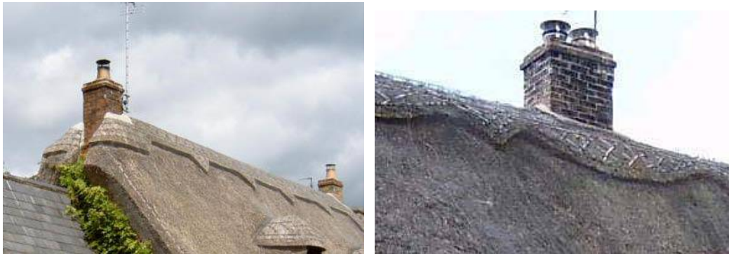
17th c. chimneys are rectangular, set midway along the ridge. 18th c. chimney stacks are usually square and built off the gable ends.
