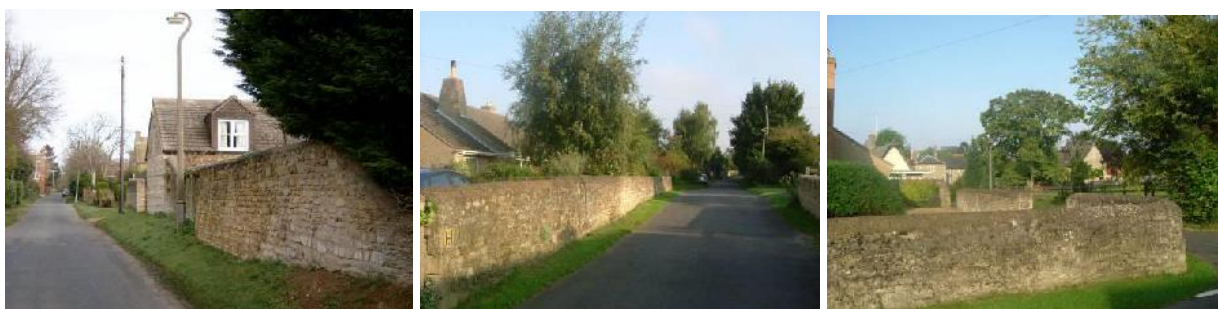
Walls in the townscape
